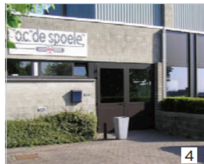
Renovaties OC Otegem
